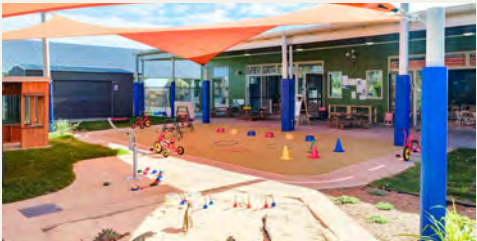
100 Public Preschools program team – recently completed preschool.
